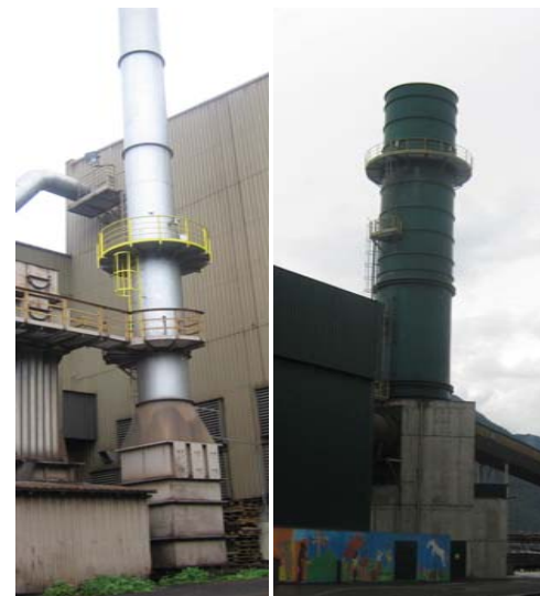
ACRONI Jesenice mokri filter PCME LMS 181 vrečasti filter PCME DT 991M
